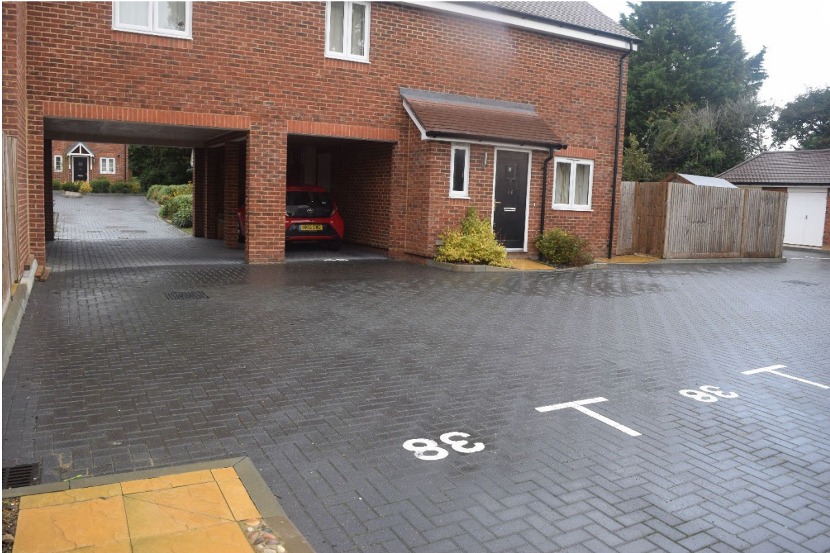
Figure 8 – Courtyard Parking to rear of dwellings, but still overlooked – Woodlands Avenue, Rowlands Castle
