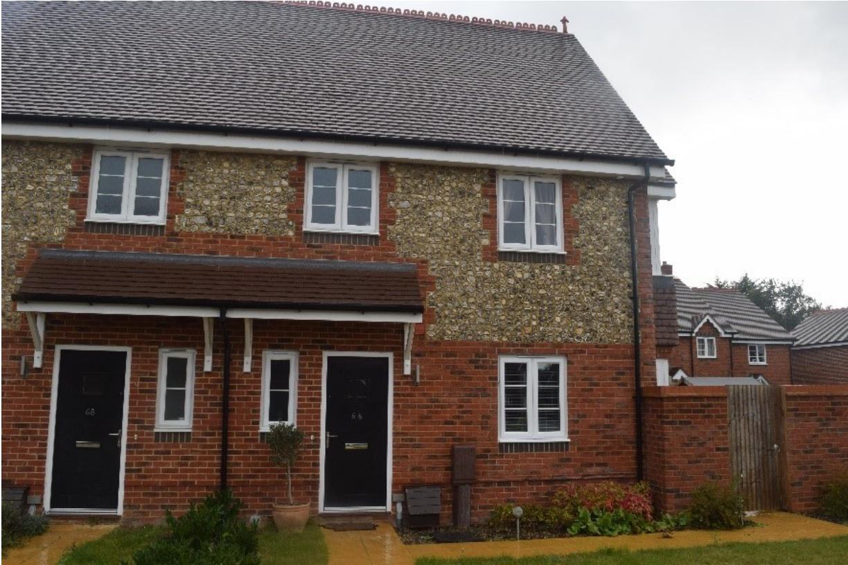
Figure 5 – brick and flint dwelling
